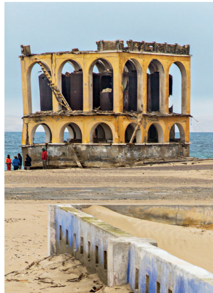
Storage. The fish oil that was produced on the island was kept in large tanks in this building near the beach, from where it was shipped. The oil was heated in the tanks to make it less viscous and easier to pump to the ships' tanks.
